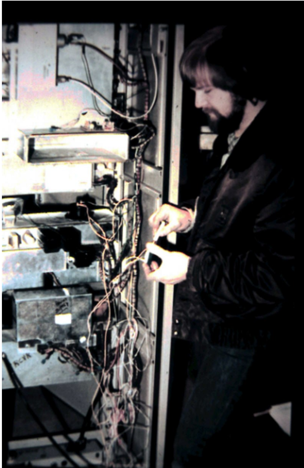
Fall, 1983 - Building the "new" DRC Motorola Motrac 147.33 repeater / Woody, w0ui
