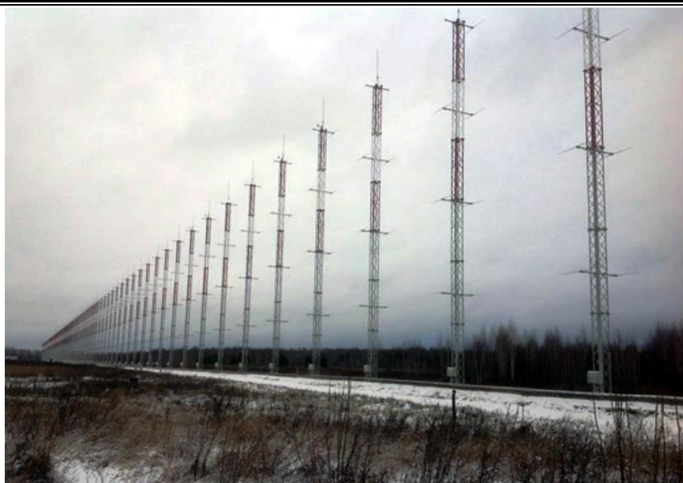
Figure 2 - A Container (29B6) OTHR receive antenna
