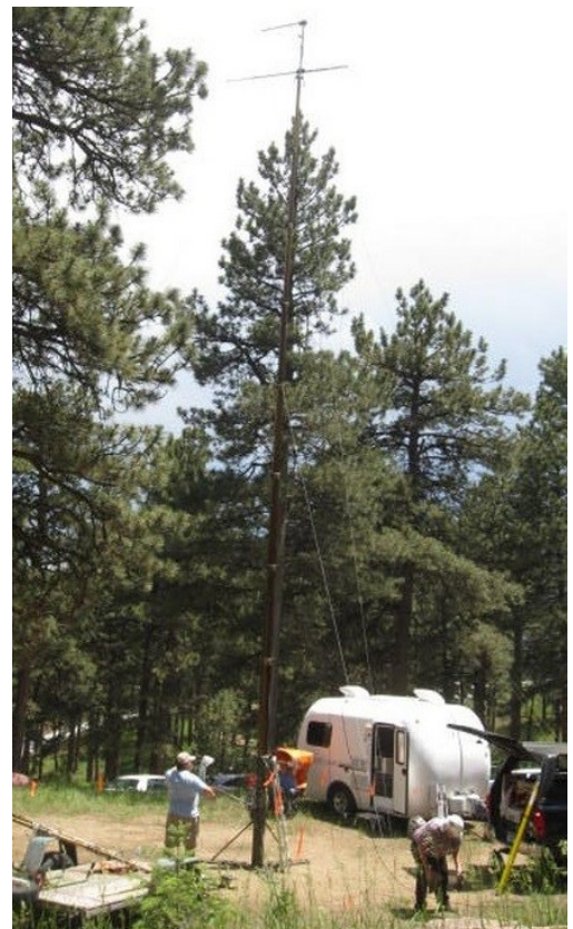
The Orlen Mast is almost set up
