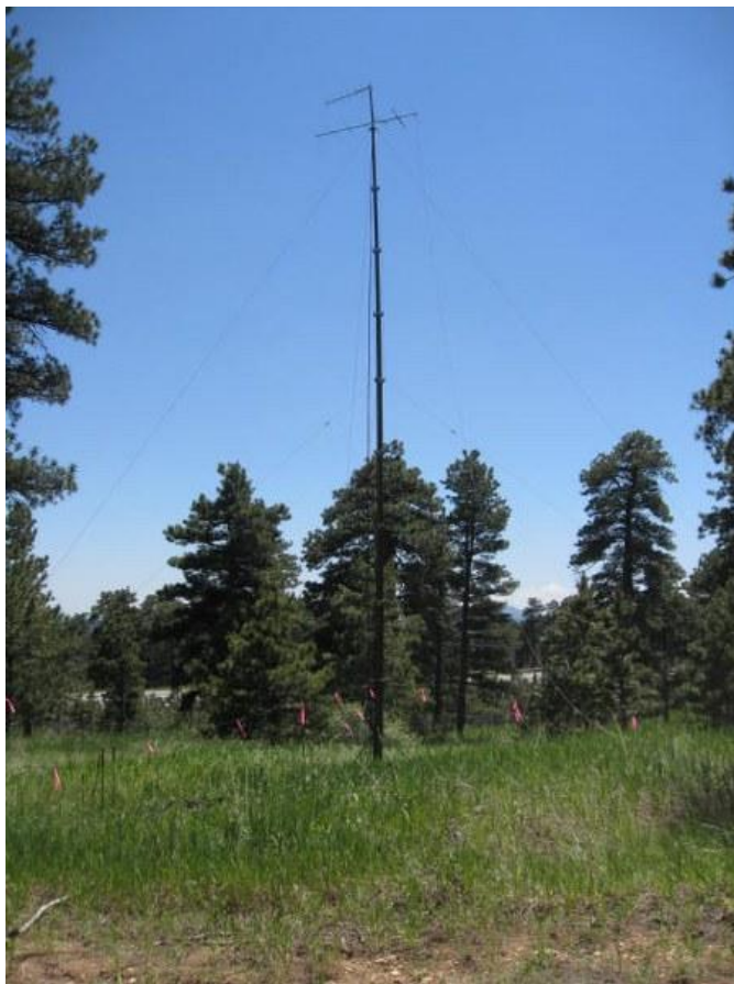
Telescopic Mast with UHF & VHF Antennas
