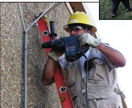
Here K0HTX is drilling a coax feed through hole.
