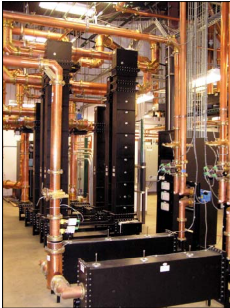
This photo shows the black band pass filters used to isolate the various TV channels. Unlike the "old" analog TV days, the digital transmissions can be on adjacent channels.
