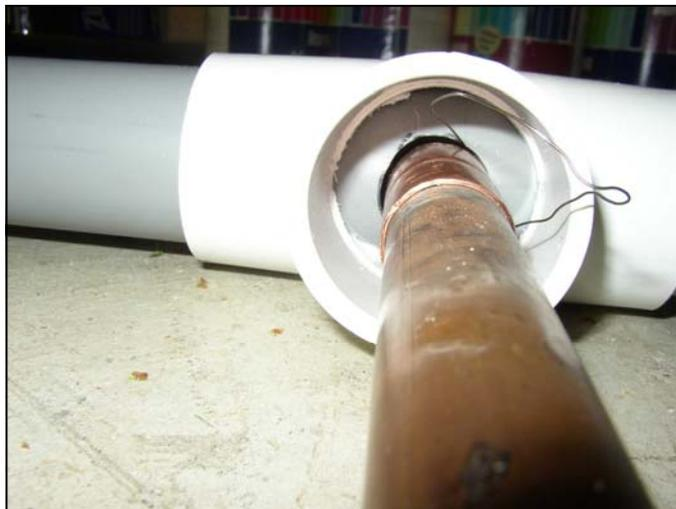
This photo shows the bottom support with the control wire being threaded down the inside of the main vertical support.
