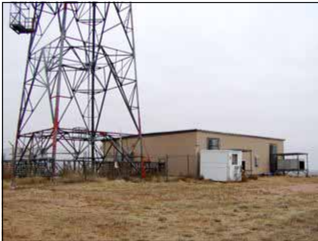
New Repeater Site Building
